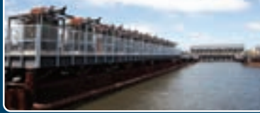
Lake Pontchartrain Pumping Station
